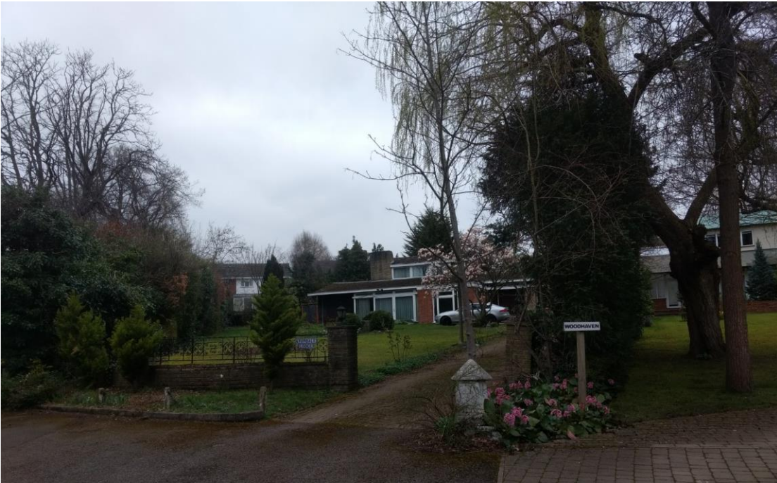
Front elevation from adjoining highway
